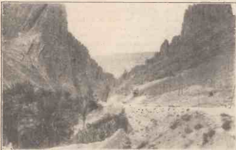
The famous gorge of El Kantara, showing the railway tunnel
