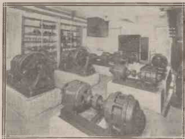
The duplication of transmitting plant to guard against interruption of the service by break-down is a subject which 2LO's recent misfortunes render of considerable interest. These are the duplicate generator sets at KGO, California.
