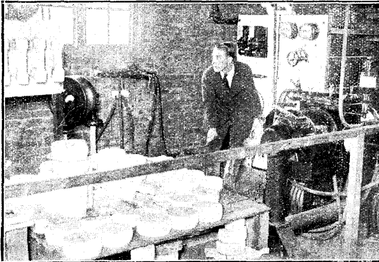
Steady progress is being made in the erection of the new high-power Post Office station at Rugby. The photograph above shows an engineer engaged in testing the aerial insulators.
