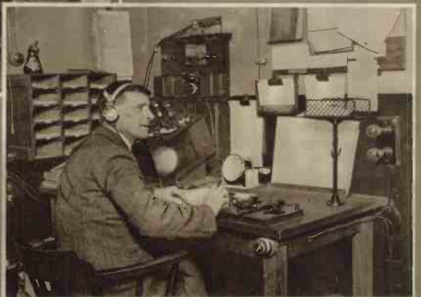
On the right: Transmitting the observed direction to an enquiring ship.
