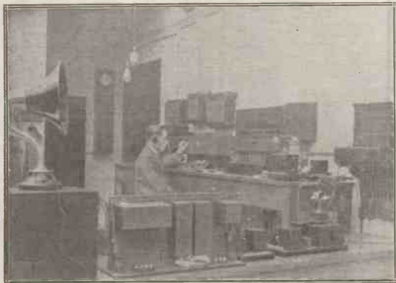
The control room at the new Belfast broadcasting station.
