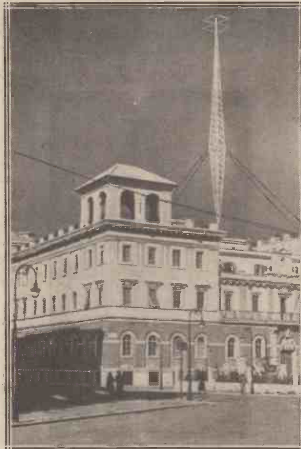
This is the studio centre of the South Italian stations. Note the anti-fading aerial of the Rome III transmitter. In this building the Italian television developments and experiments will probably be carried out.
