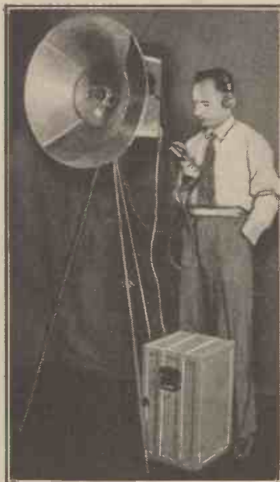
A combined Telefunken micro-wave transmitter and receiver for two-way communication. The same aerial and reflector are used for both transmission and reception.
