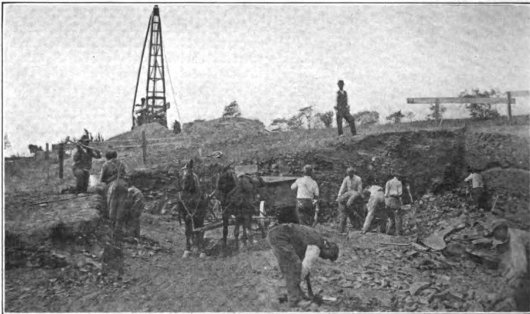
Rapid progress is being made with the excavations for the transmitting station at New Brunswick.
