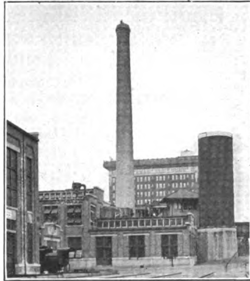
On this 175-ft. brick stack at Scranton, Pa., will be suspended an antenna about 700 feet long.
