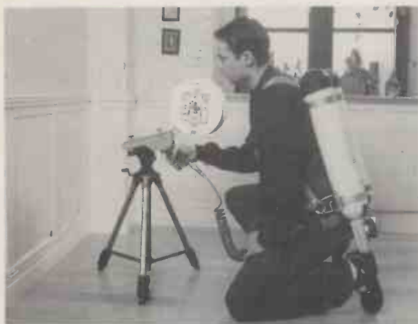
Ultimate connection... The final winner in broadband-to-the-home will be fibre optics – replacing xDSL, cable modems, satcomms, and terrestrial broadcast, it is claimed. Ericsson Cable’s Ribbonet system (pictured) can inject optical cables into existing cable conduits.
