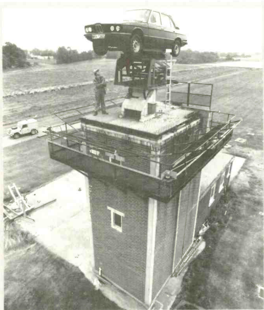
As part of British Telecom's remit to diversify, the research people at Martlesham have come up with a possible solution to the capital's parking problems. And if that doesn't work, they'll use the system to test cellphone aeri-als.
