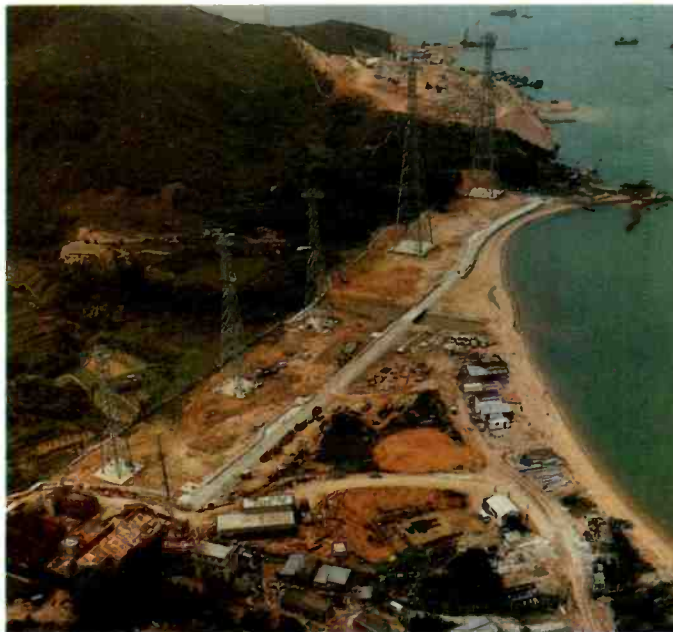
Under construction: a new BBC relay station at Hong Kong.
