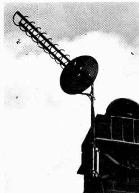
Helical aerial prototype erected on site.
