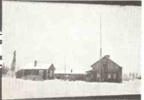
The 70ft. wooden aerial mast at the main station, a typical Lapland log cabin.
