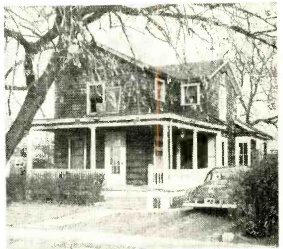
Fig. 2. Outside view of house. Entrance door to living room is at right rear of porch. Second unwanted door is behind glass-pannelled storm door at front.
