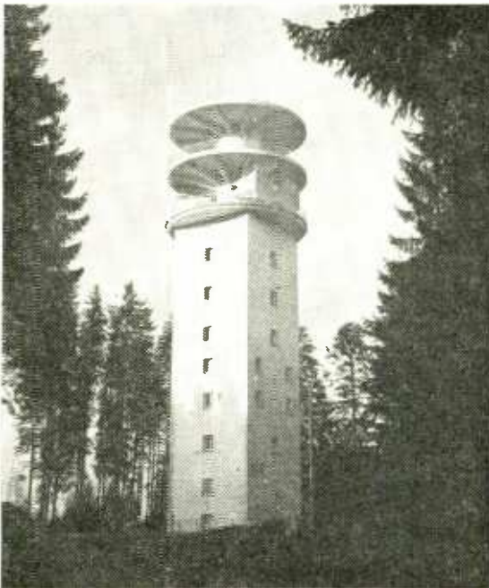
Television relay station in the Paris-Strasbourg chain at Dabo la Hoube in the Jura, constructed by Cie Generale de Telegraphie Sans Fil.
