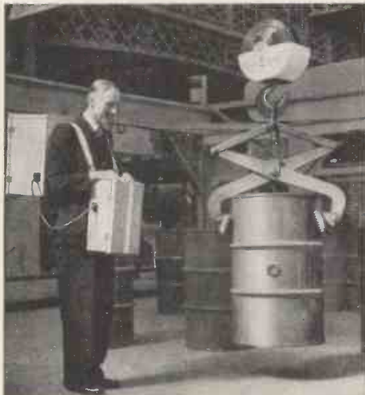
For the precision handling of bulky, cumbersome or dangerous loads (such as toxic chemicals or explosives), and for assembly operations where the crane hook may be out of sight, radio-controlled equipment is frequently used. This picture—from a recent issue of MECHANICAL HANDLING—shows the system in operation.
