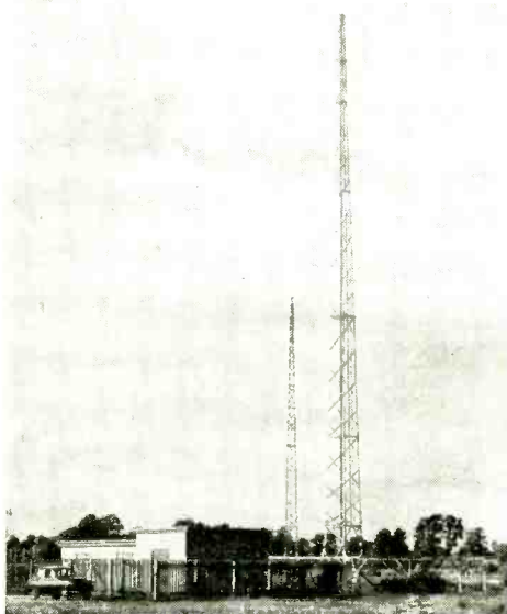
Below: Fig. 6. Aerial installation for a fan marker. These operate on a frequency of about 75½ Mc/s.
