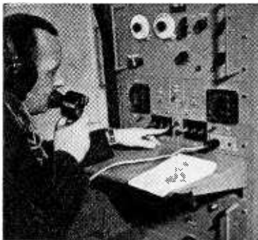
CONTROL PANEL on the Ekco E.H.F. airport installation at Southend. Transmitters and receivers are above the writing shelf and all power supplies are below.
