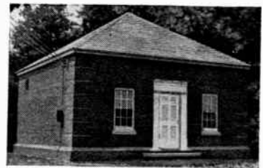
[Courtesy: Bell System Technical Journal.] Fig. 2. Auxiliary repeater station on New York-Philadelphia route.
