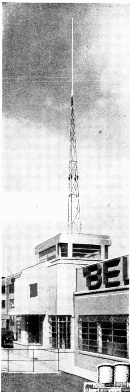
The illustration above shows the Belling-Lee Skytower Aerial—a 35 ft. lattice mast surmounted by an 18 ft. Skyrod.
