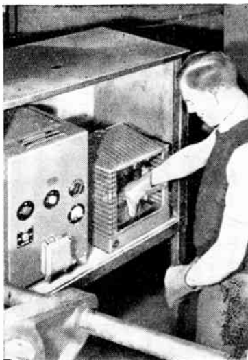
A comparatively simple case of effective anti-interference screening: the "work" chamber of a Rediffusion \frac{1}{2} kW heater, mounted close to the generator and fully screened.
