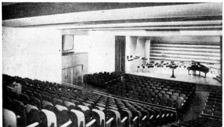
SOUND REINFORCING is employed in one of the rebuilt broadcasting studios of the National Broadcasting Company in Radio City, New York. The small console incorporating the controls is located in the seating section. The sound reinforcing system is used to permit studio audiences to hear those broadcast artists who perform close to the microphone, and would, therefore, be inaudible to a large section of the audience.
