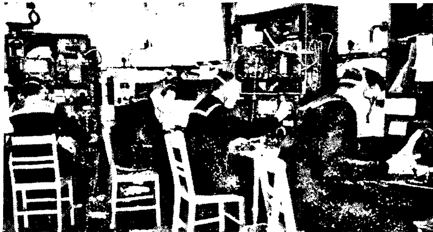
THE BATTLE OF THE ATLANTIC. One of many such wireless rooms at various points along our coasts where communication with convoy escorts is maintained. Each telegraphist is operating a transmitter and receiver of which there are several at each station. The transmitters, some of which are of considerable power, have a very wide range.
