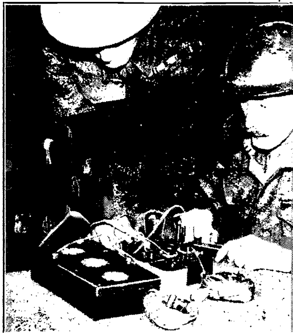
The transmitter unit, batteries, aerials and accessories are distributed between two leather carrying cases.
