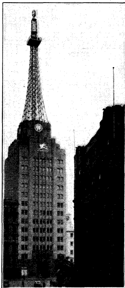
The Pegasus crest of Amalgamated Wireless of Australasia stands out prominently on the façade of the new A.W.A. building in Sydney. The 165ft. steel tower brings the overall height of the structure, which is the highest in Australia, to 365ft. The broadcasting station 2CH will eventually be housed on the two top floors.
