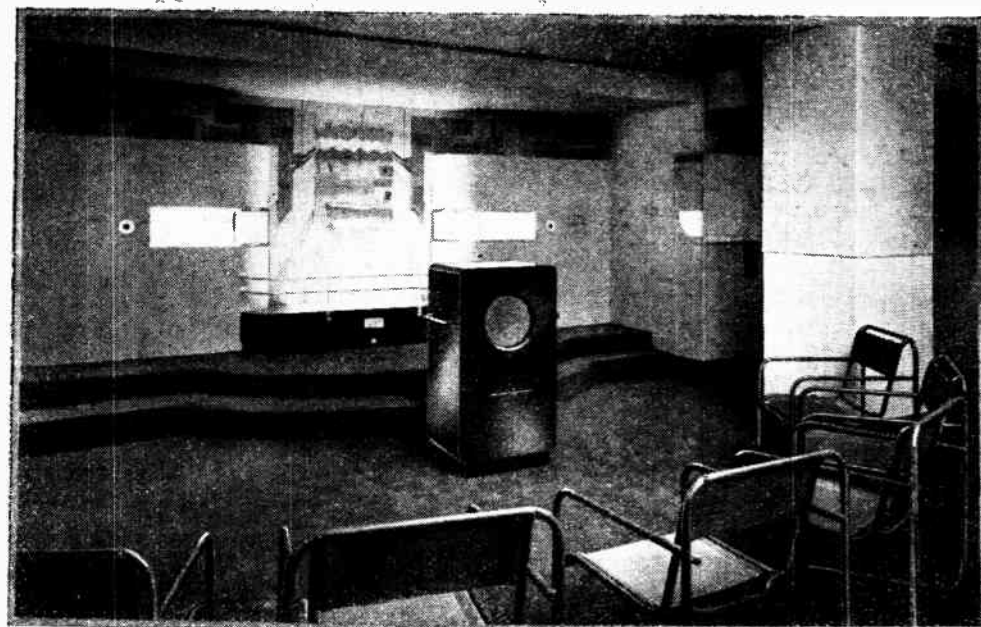
The interior of one of the listening rooms at Broadcasting House, the headquarters of the B.B.C., where great care has been taken to provide realistic reproduction.
