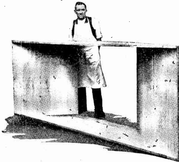
Fig. 3.—The final wood section. This is lined with sheet metal to preserve a uniform surface within the sound conduit.
