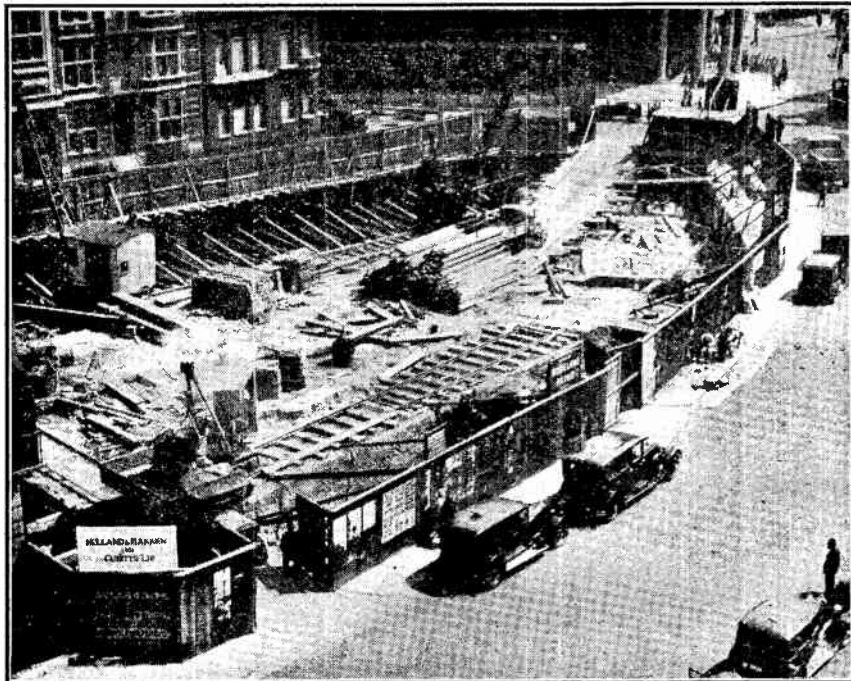
FUTURE HOME OF BROADCASTING. Work has now begun on the erection of Broadcasting House, Portland Place, London, W. The photograph shows the preliminary excavations in progress. Part of the Queen's Hall can be seen in the background on the right.
