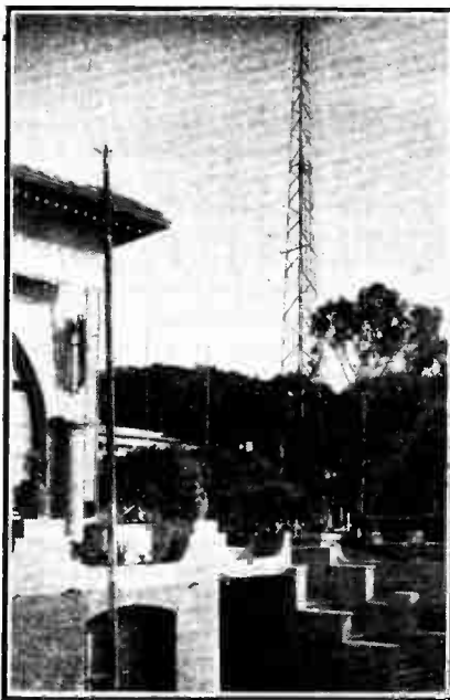
WHERE THE SUN STILL SHINES. A glimpse of the Juan les Pins broadcasting station at Nice, which sometimes can be heard in England, though the power is only 0.5 kilowatt. The wavelength is 245 metres.
