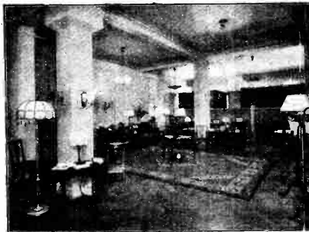
A PERMANENT WIRELESS SHOW. A corner of the new wireless and electrical showroom of the B.T.H. Company at Crown House, Aldwych, London, W.C.
