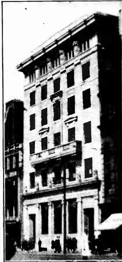
"BROADCASTING HOUSE." The new Manchester headquarters of the B.B.C., known as "Broadcasting House," in Piccadilly. Structural alterations are now in progress, and include the provision of a large studio with a gallery for the audience.
