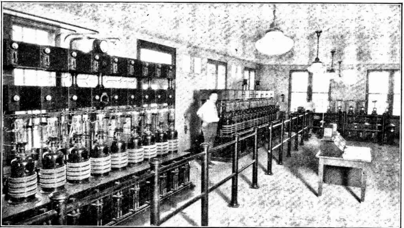
General view of valve panels: on the extreme left, the radio-frequency amplifier; in the centre, the modulator; and on the extreme right, the high-power rectifier.
