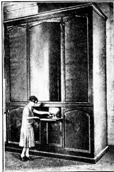
Fig. 1.—Gramophone reproducer with 20ft. horn capable of reproducing frequencies down to 40 cycles.
