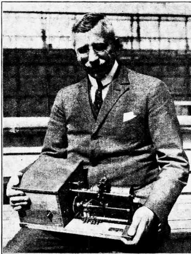
WIRELESS PICTURE RECEPTION AT SEA. Prof. Max Dieckmann with the radio picture receiver with which he had been conducting experiments in the s.s. "Westphalia." Weather charts transmitted from Hamburg Observatory were received successfully and displayed on board ship.
