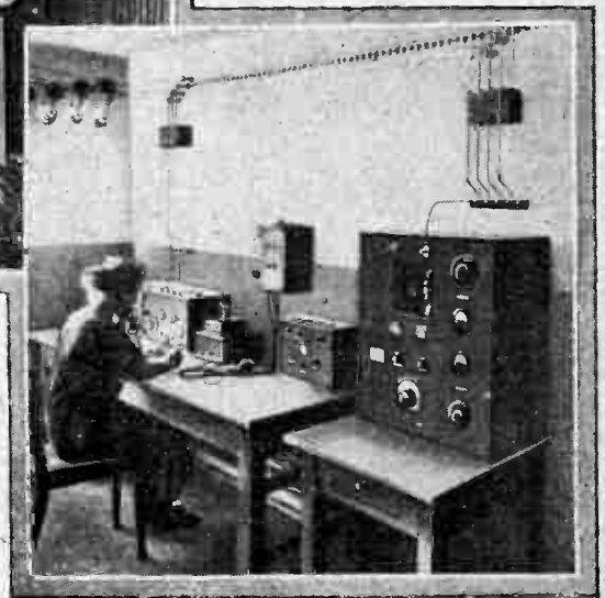
View of the wireless equipment in a railway telephone exchange.
