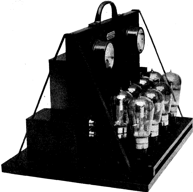
Fig. 1. The "C" Amplifier with eight L.S.5A valves in parallel.
