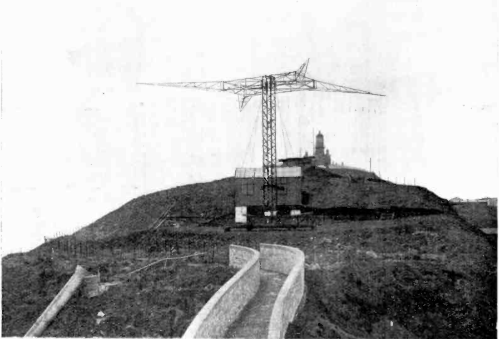
Fig. 106. The Parabolic Reflector at Inchkeith, Firth of Forth, Scotland, as used for directional short wave wireless telephony.
