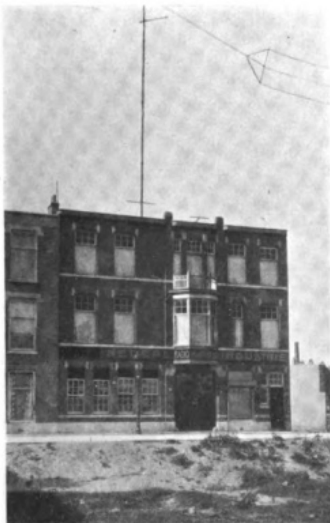
Fig. 1. Front view of the Works of the Nederlandsche Radio Industrie at the Hague.
