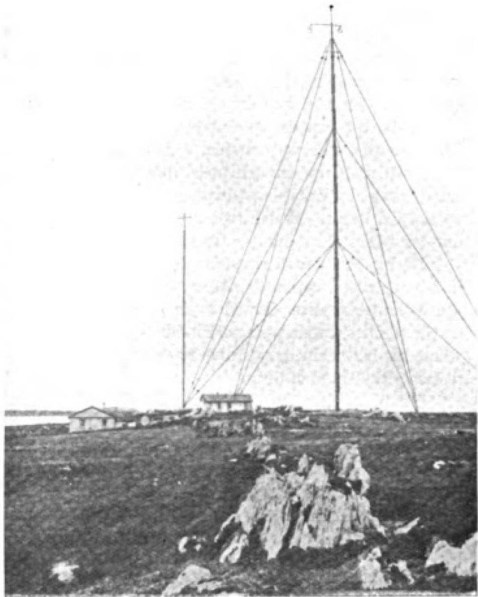
THE TWO STEEL MASTS AND STATION BUILDINGS.
