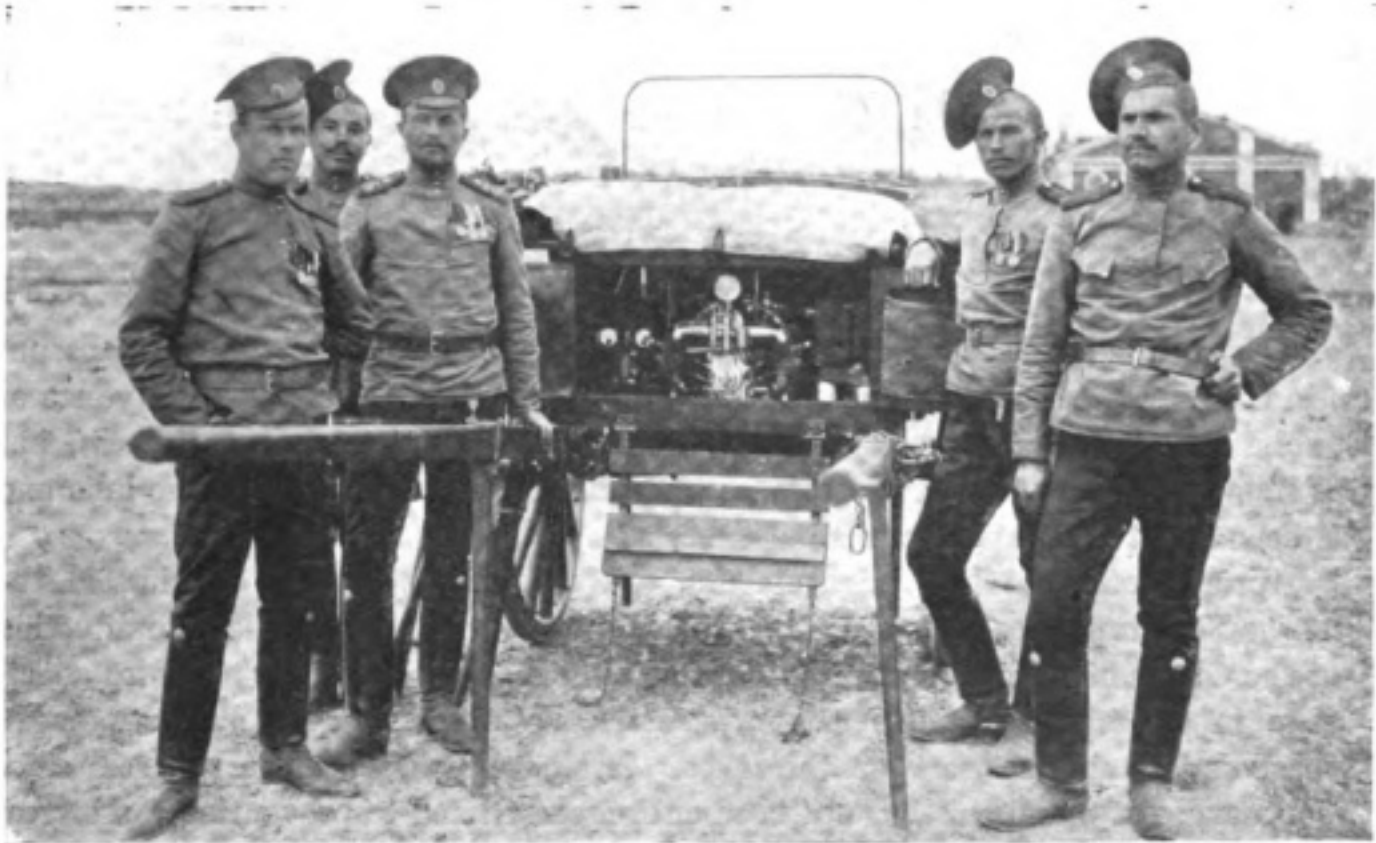
RUSSIAN PORTABLE WIRELESS APPARATUS. MANY OF THESE STATIONS ARE WORKING IN CONJUNCTION WITH THE ROUMANIAN SETS SHOWN ON THE PREVIOUS PAGE. THE ABOVE ILLUSTRATION SHOWS THE PETROL ENGINE CONNECTED TO THE TRANSMITTING DYNAMO.
