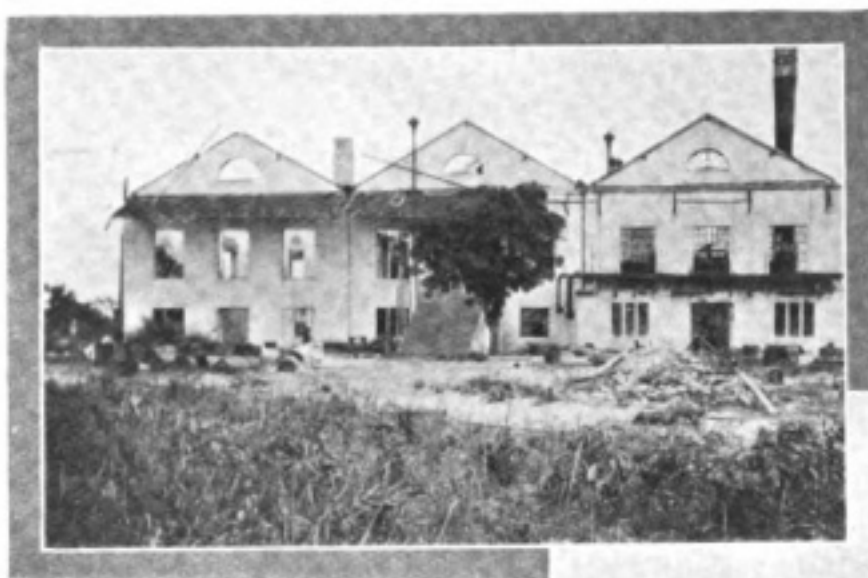
REMAINS OF POWER HOUSE, KAMINA.
