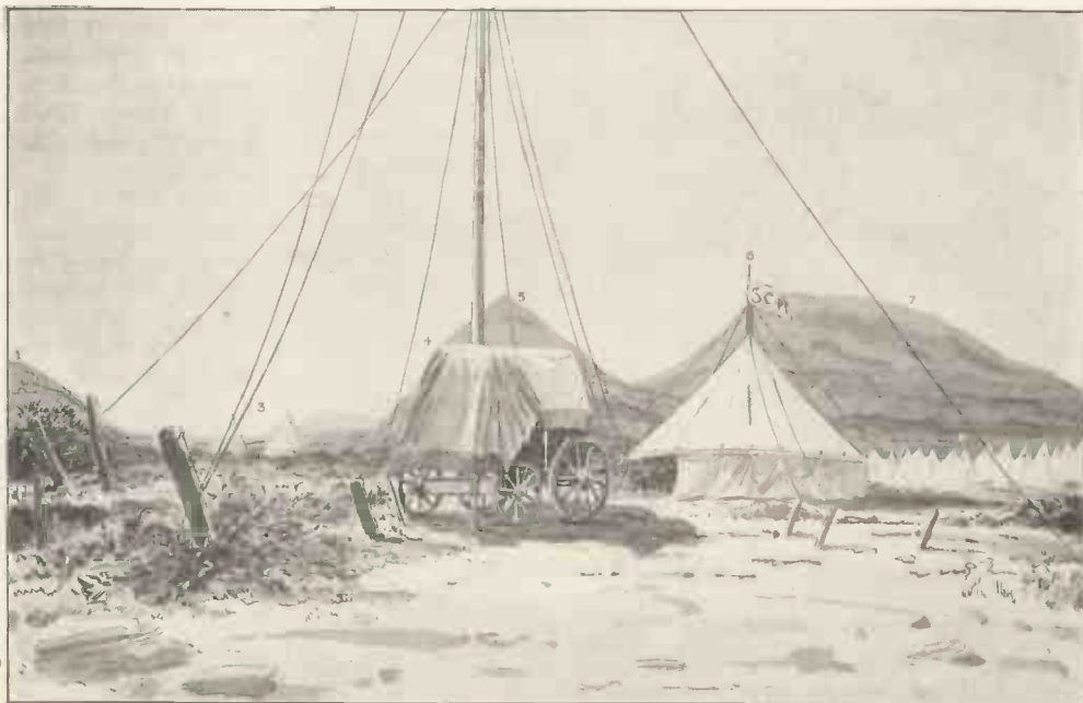
1, Camp Kopje. 2, Pit for Wireless Balloon. 3, Wireless Camp. 4, Wireless Wagon and Mast. 5, Sharp Kopje. 6, Soldiers' and Christian Association Tent. 7, Big Kopje.
