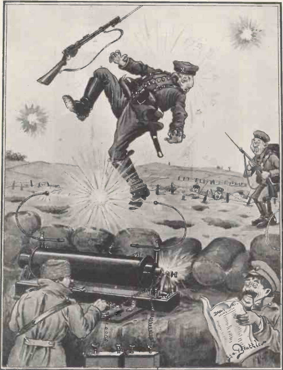
Wireless Entanglements for Trenches.
