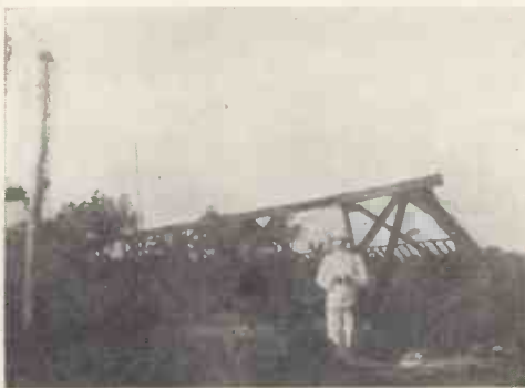
The Fallen Wireless Tower at Duala.
