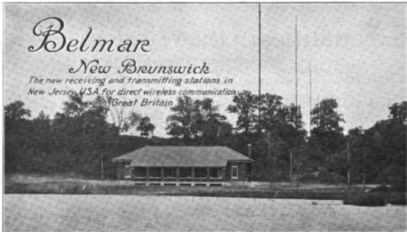
Operating Building at Belmar.
