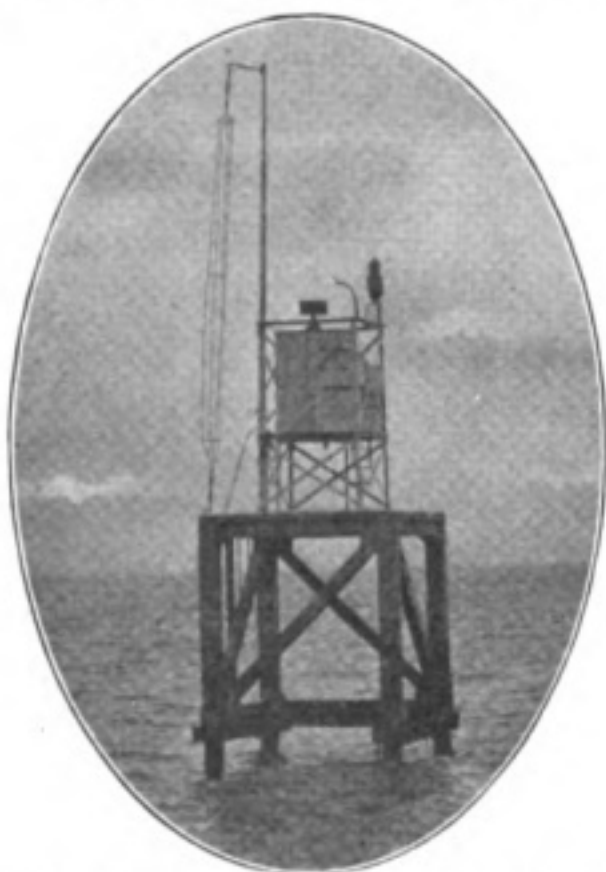
Wireless Fog Signal at Roseneath Patch (Clyde).
