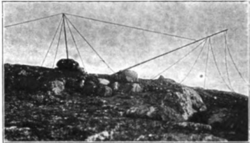
Raising the new mast at Cape Harrison.
