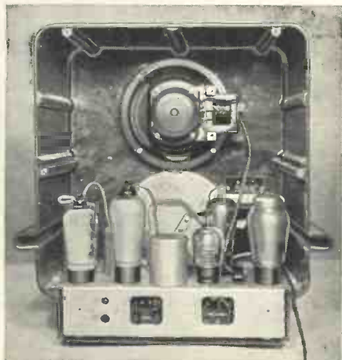
"A three-point tone control is fitted at the back of the chassis . . . delayed automatic volume control is another of the high lights"
