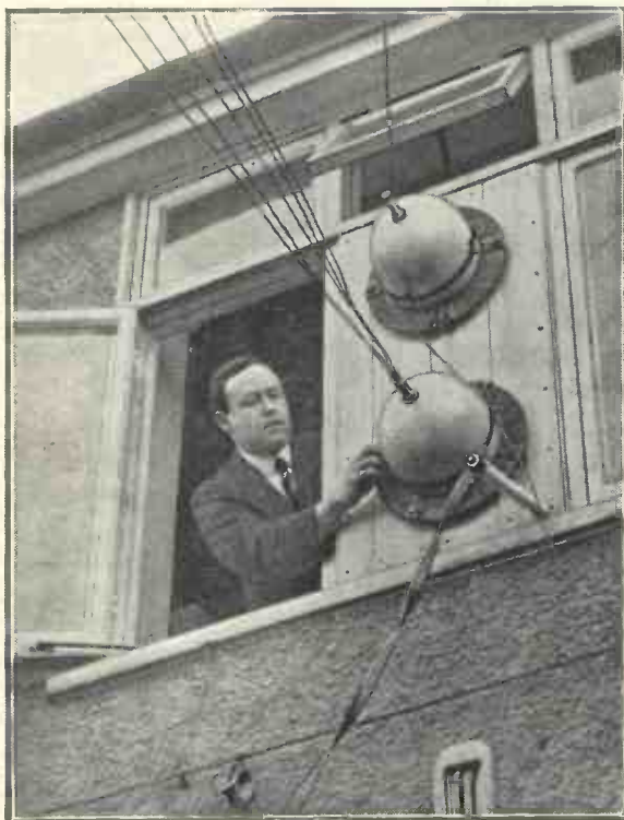
AERIAL USED FOR TRANSATLANTIC TRANSMISSION The heavily insulated lead-in of the aerial used by J. L. Baird on the occasion of his Transatlantic television transmissions in 1928
