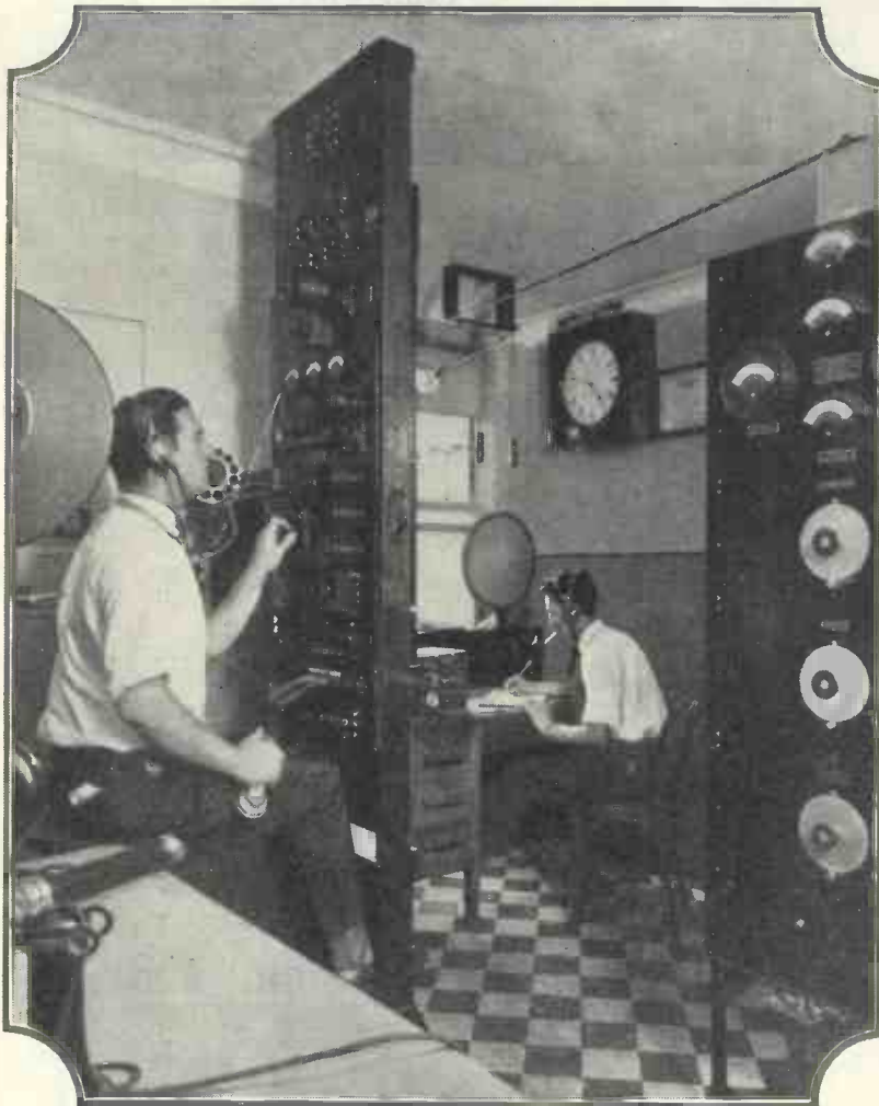
INSIDE AN AMERICAN BROADCASTING STATION
