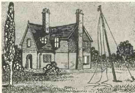
Unfortunately before the guy ropes were secured . . .
