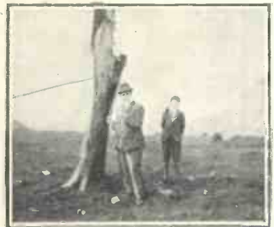
Holding the aerial hoisting string
