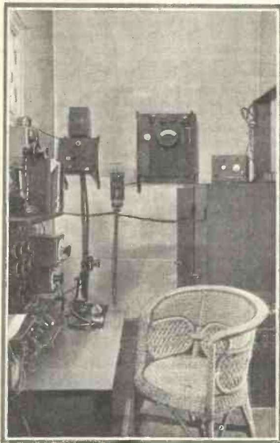
Control room at CKAC, owned by La Presse.
