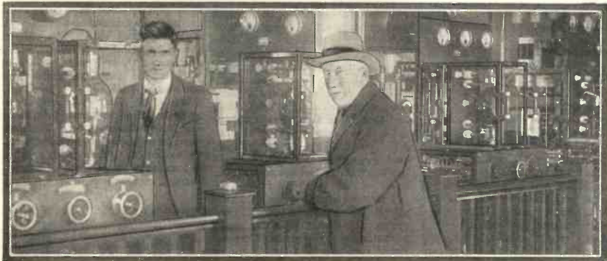
At the Dublin broadcasting station. Leaning on the rail is Mr. Mulligan, Chief Engineer of the Irish Free State Post Office.
