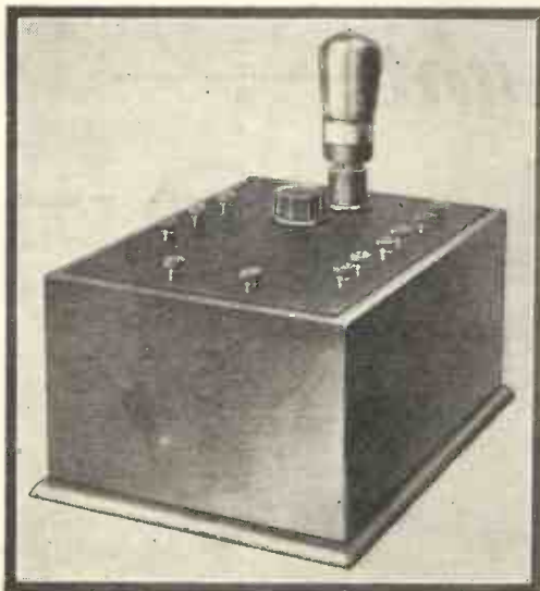
Completed One-valve Amplifier.
