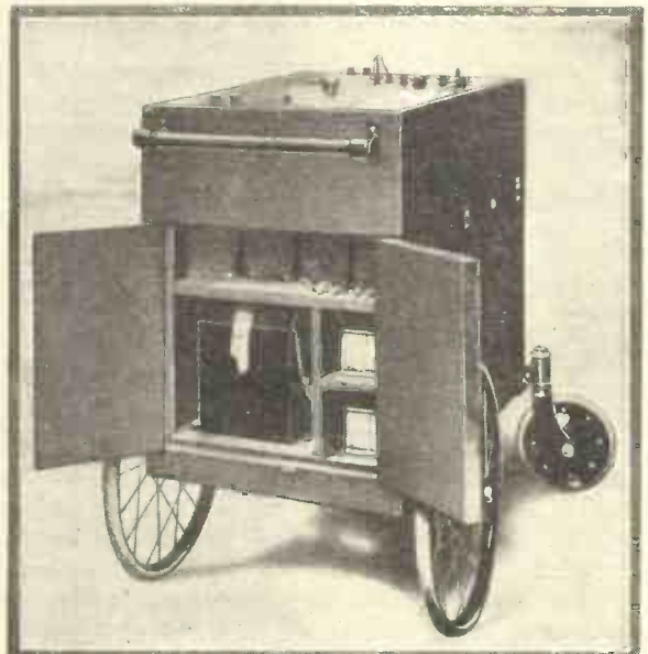
Battery Accommodation in Portable Stethophone.
