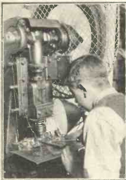
The blank for the anodes are first stamped out and then pressed to shape.
