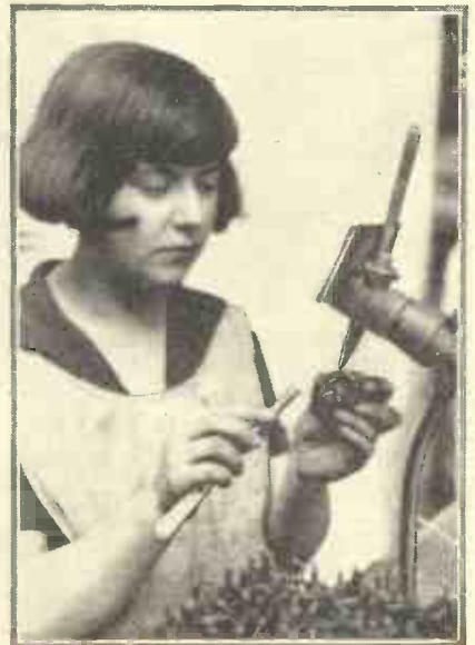
The lead wires are soldered to the legs by means of a gas-heated bit.
