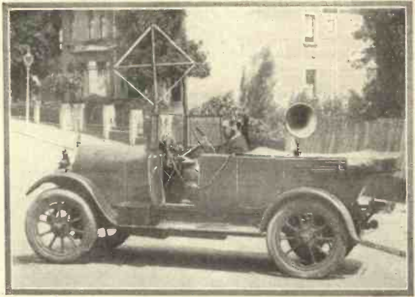
Working a Loud-speaker with a Three-valve Reflex Set
